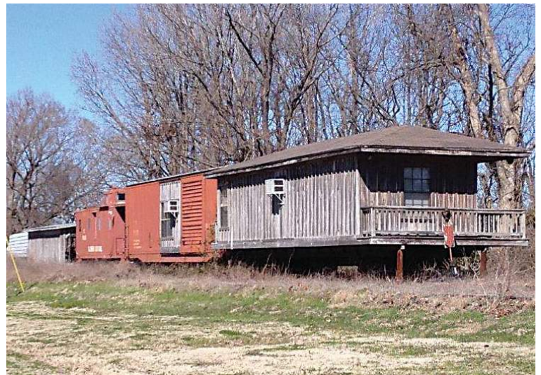
This house in Issaquena County made of a train caboose and box car shows the resourcefulness of Delta residents in making a place to live.
